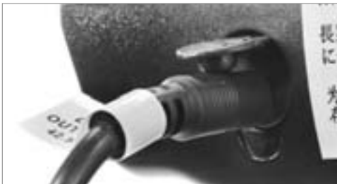
Charging the battery
